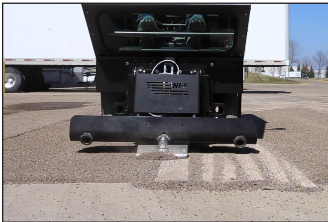
Machine scraping epoxy-covered concrete.
